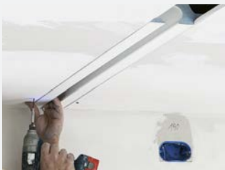
Fix article onto false ceiling using screws.
