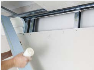
Apply adhesive on the surface to be glued after making the hole.
