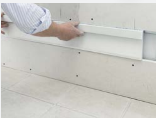
Fix article on metal structure using screws.
