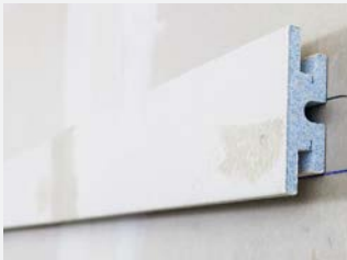
Plaster over screws.
