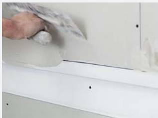
Apply plaster in three layers.
