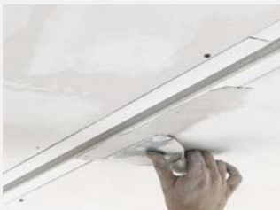
Apply plaster in three layers.
