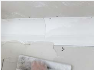
Apply plaster in three layers.
