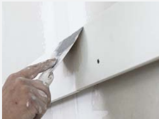
Plaster along joint between the two profiles.
