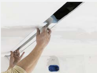
Insert article in false ceiling hole.
