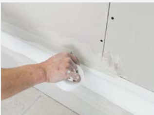
After applying second layer, lay mesh tape.
