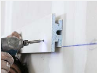
Fix article using screws.
