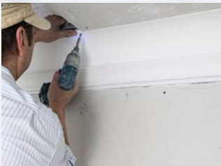
Fix article on metal structure using screws.
