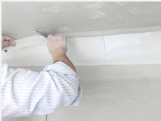
After applying second layer, lay mesh tape.
