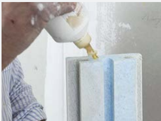
Apply adhesive also on article head if two profiles are to be glued together.
