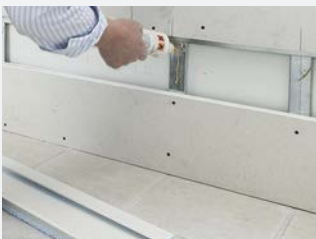
Apply adhesive on the metal structure.
