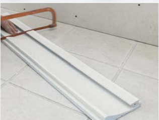
Use a hacksaw to cut article to measure.
