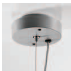
Ceiling rose with supporting and power supply cables.
